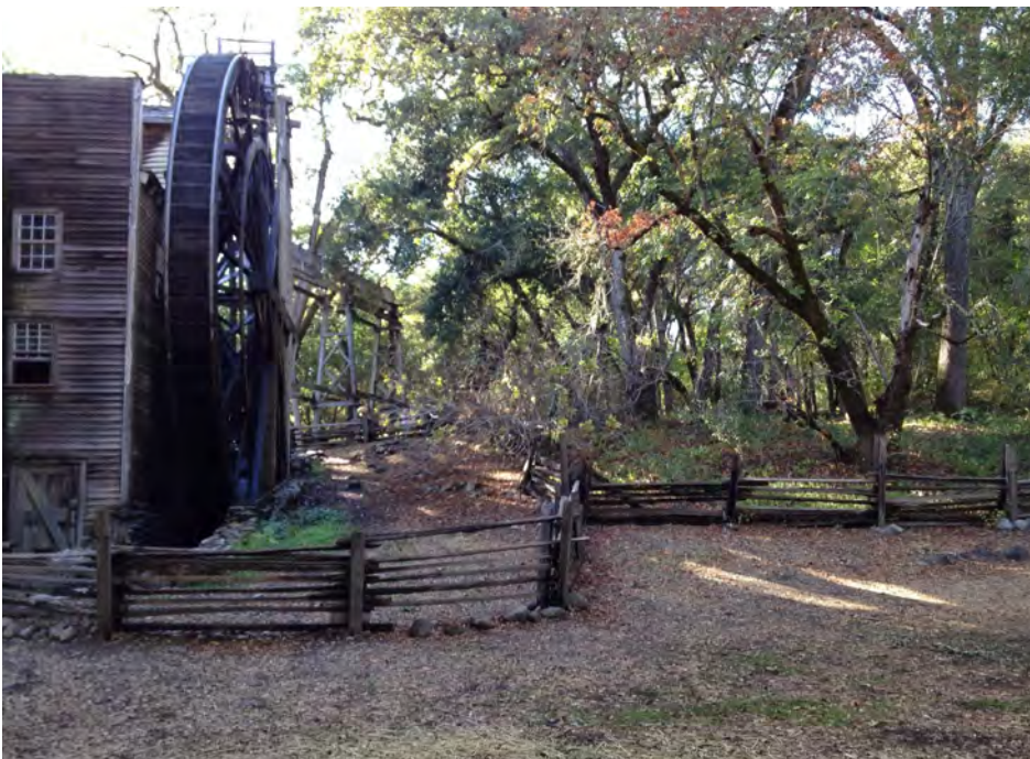
Napa Valley Grist Mill historic site is built across 2m-high scarp of West Napa fault.
